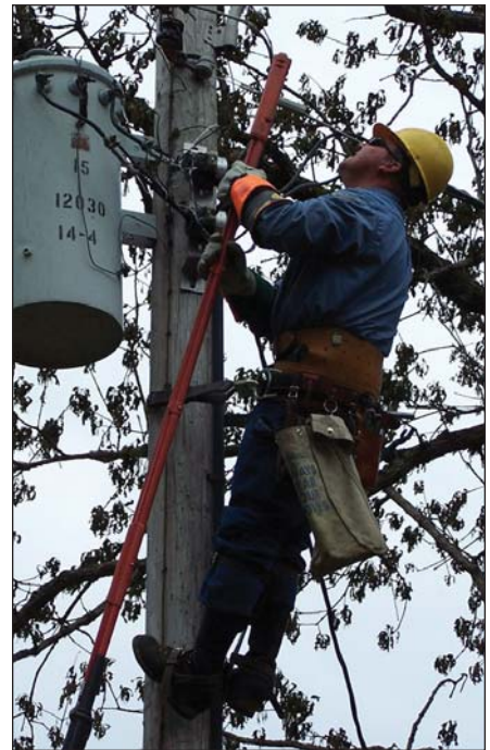
David Tacker disconnects the neutral to make repairs.
