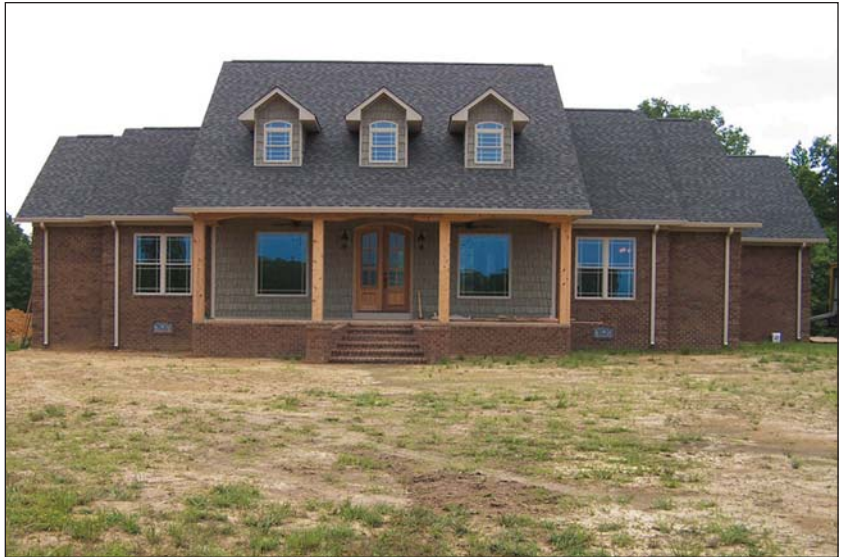
The Burkses will enjoy years of comfort in their new home with the installation of a ground-source heat pump.
