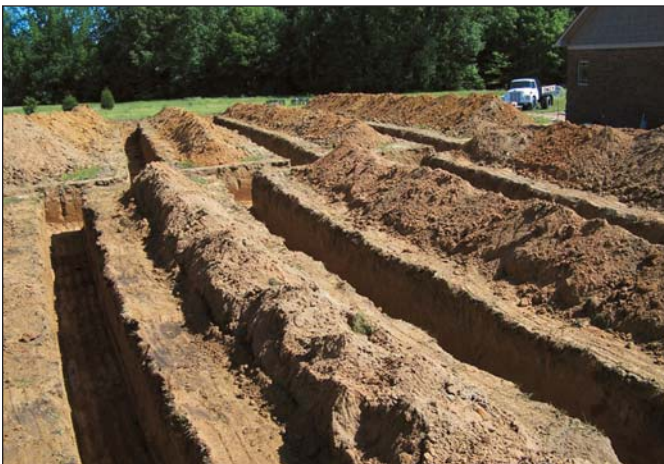
Trenching will make this system more expensive up front than traditional heating and cooling systems, but the energy savings will offset the cost in about five to six years.
