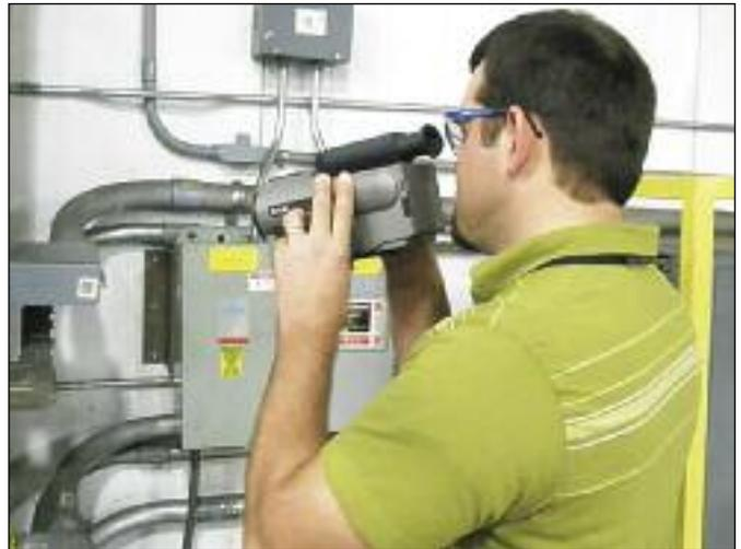
Brian Smith, TVA power utilization engineer, performs an infrared scan at Monogram Refrigeration in Selmer.
