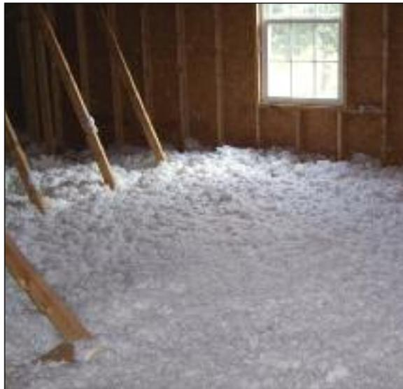
In selecting the insulation for these areas, you will need to consider the R-value. The higher the R-value, the more effective the insulation. Different types of insulation will require different depths for the same R-value, so this is something you might want to talk over with a contractor.
